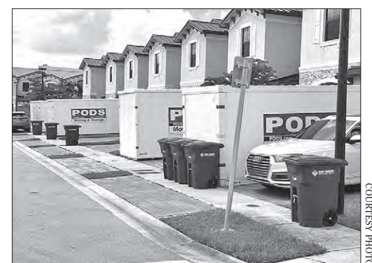
Lennar built these homes in Florida for the Seminole Tribe last year.
